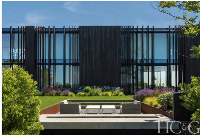
This project by BMA Architects was a runner-up at the 2023 IDAs. Photograph by Michael Stavaridis
